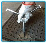
2 Use the "L" extremity as rotation cleaner to erase in the internal aperture of the slots to liberate completely the internal rotation space and allow the insertion of the key, can also be sued as lever to unlock the latch that blocks some covers before opening.
