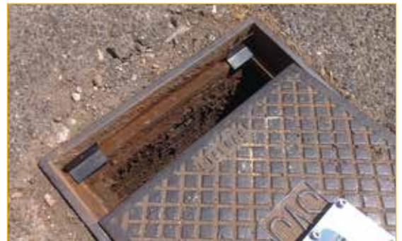
Shims positioning between cover and frame.
