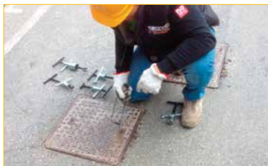
Suitable for mechanical opening of manhole covers.
