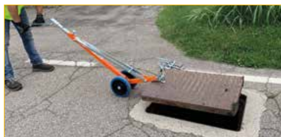
Use 3: mechanical opening with locking clamps.
